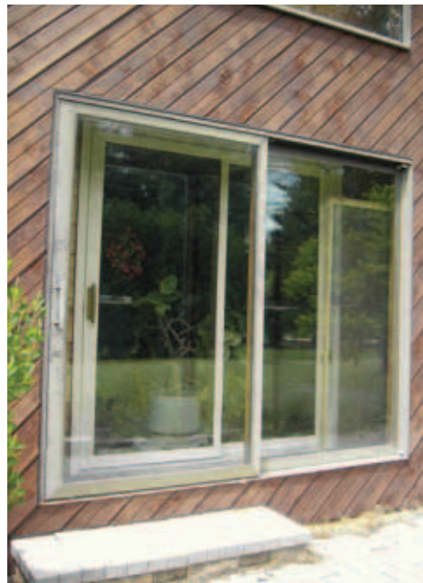
The interior and exterior walls each have their own set of windows and doors.
