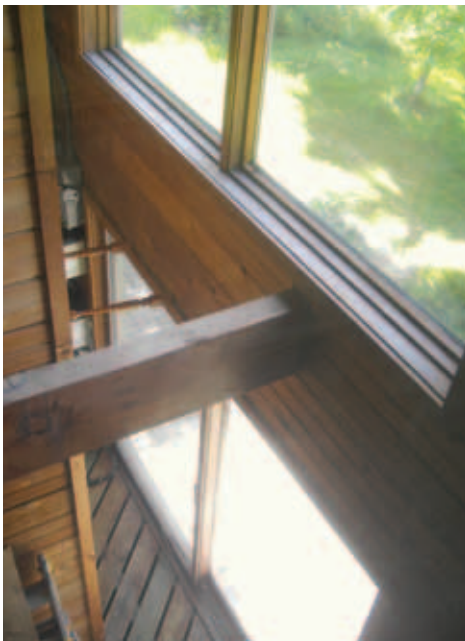
This 1981 double-walled passive solar home in Newark, DE, stays comfortable thanks to a convective loop. No fans necessary.
