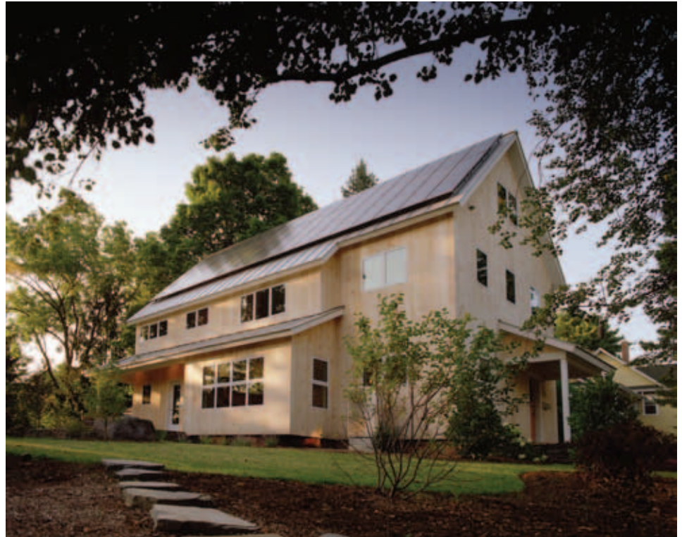
Thanks to solar renewable energy credits and the low interest rates of 2009, the Ross residence's PV system is a moneymaker.
