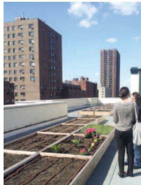
Each Lexington Ave. apartment has a rooftop garden plot with automatic trickle irrigation.
