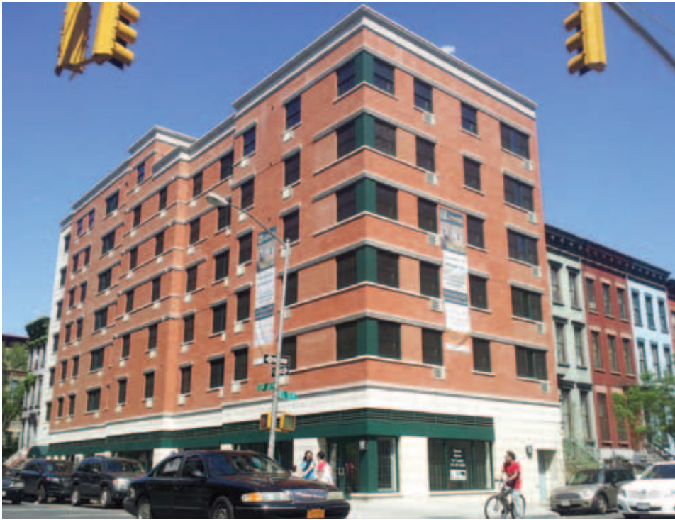
The pioneering Bluestone Organization's Lexington Ave. co-op is among the first in New York City to be constructed with insulated concrete forms.
