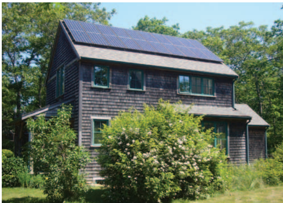
The 4.76 kW PV system far exceeded expectations; the surplus for the year could be used to run an electric car over 10,000 miles.
