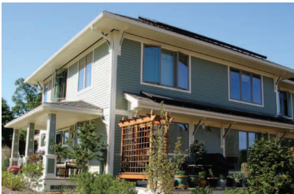
The Wright home is equipped with a 6 kW PV system, which typically yields a credit on the electric bill, despite an air-source heat pump, an electric heat-pump hot water heater, and an ERV.
