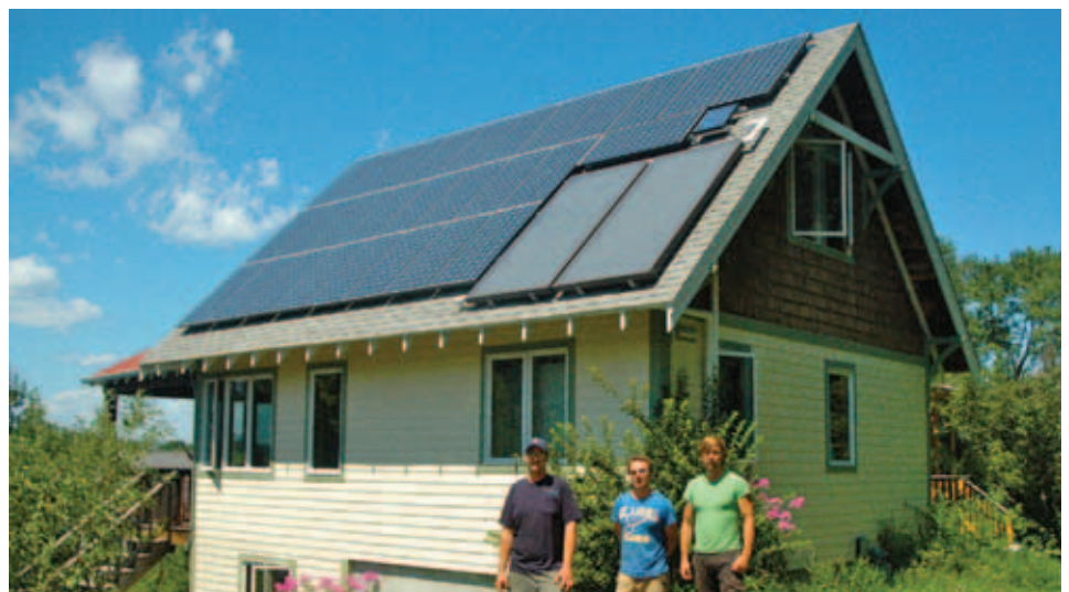
A 6 kW PV system drove the Kraus-Fabel residence to net zero. "Having no energy bills has been great," says Mary Kraus.
